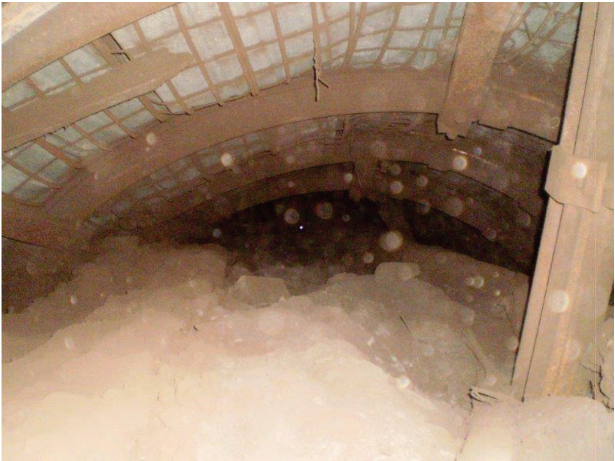
Fig.8: Drift totally collapsed
