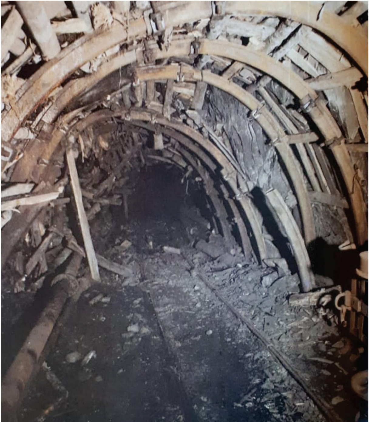
Fig.7: Lower drift steel set and wood support, heavily damaged
